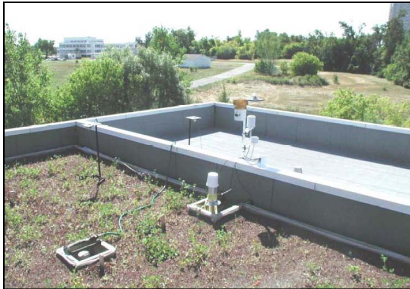
Figure 5.1 Canadian study photo showing the data collection surfaces of each roof.
